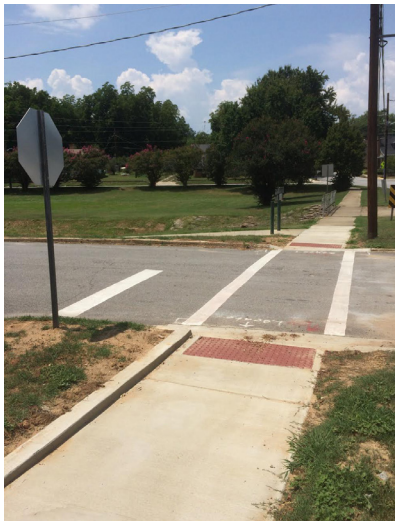
Figure 6. Newberry, SC sought to improve ADA accessibility and connectivity in a low-income neighborhood. Signage and paint were budgeted for crosswalk improvements, which were installed by the SC Department of Transportation (SCDOT). It is important to engage SCDOT staff early in the process since they know what permits are needed.
